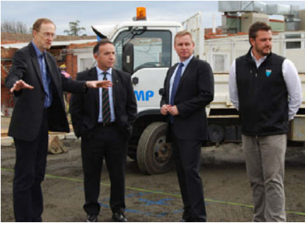
Bass MP Andrew Nikolic joins Minister Rockliff (right), Dr Main (far right) and Dr Carson (left) on a tour of the construction site
